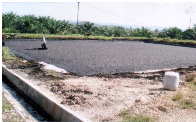
Fig. 7. CPO liquid reservoir was settle became the solid sludge. End of reservoir its waste was settle during 30 days, than it possible to use as fertilizers
